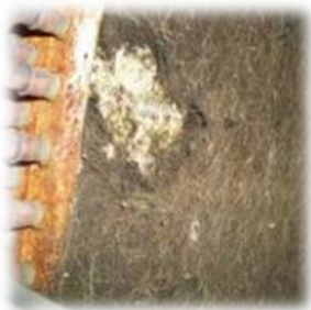
Evaporator plugged with hair
