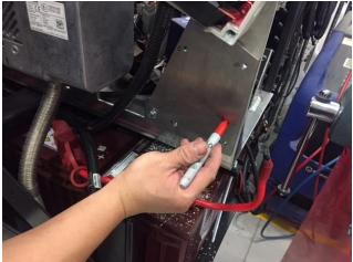
7. Remove mounting plate and drill out marked holes (1/4") on frame
