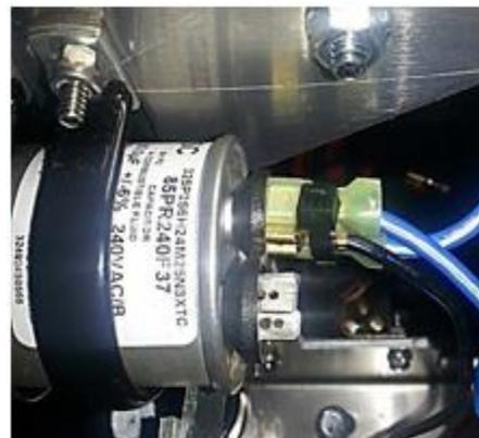
Tie strap in place on the first set of run capacitor terminals. It contains two blue wires and a black wire from the start capacitor.
