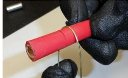
7. While holding wire position cross the wires near insulation to allow twisting room.
